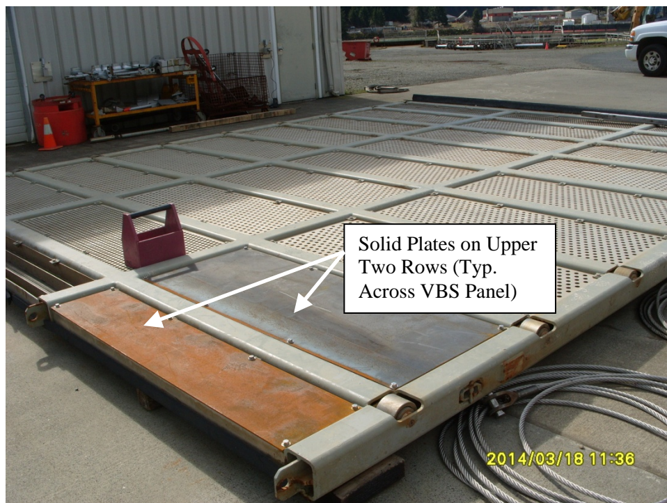
Figure 31. VBS in Process of Being Modified
